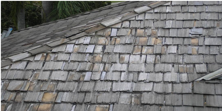
Photo 8: Wood shakes roofing
