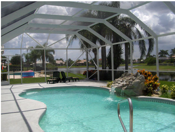
Figure 1 – Typical Screen Enclosure
